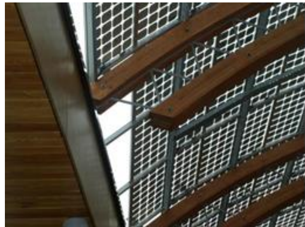
EXAMPLE OF GLASS ROOF WITH PV MODULES (Source:SEC)
