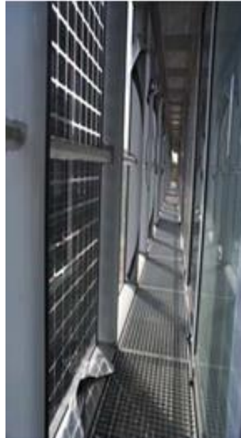
BIPV IN COLD FAÇADE (Source: SST)
